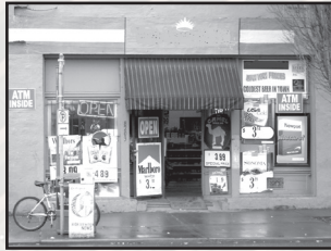
A would-be criminal may see this store as an easy one to rob because ads in the windows almost completely obscure the view inside.
