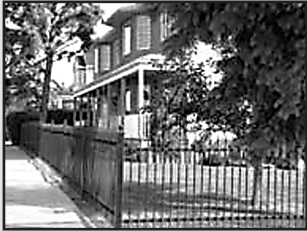
The fencing defines the site, thereby controlling access to the property. It also allows for strong natural surveillance.
